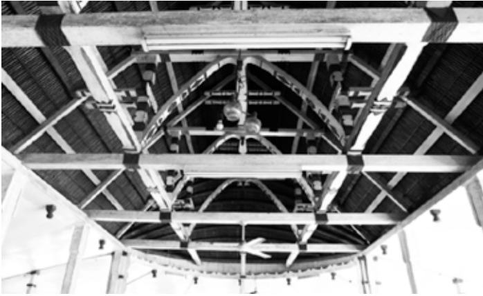
Figure 5: Interior Roof Space of Maota Lepea (photograph by the author).
