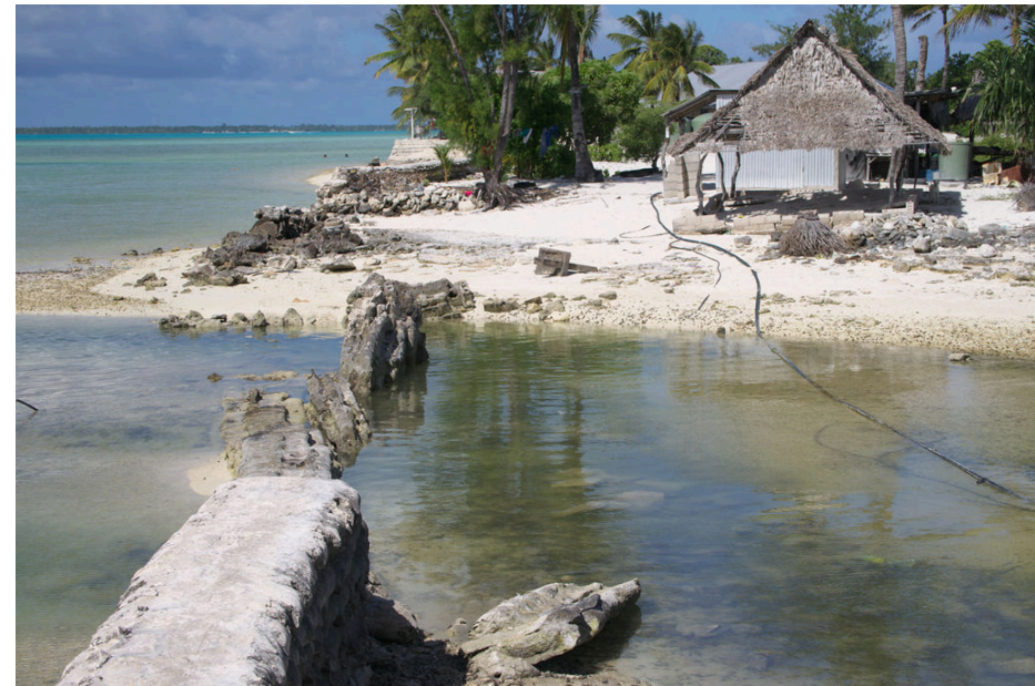
Damaged seawall, Bikenibeu, Tarawa, Kiribati
