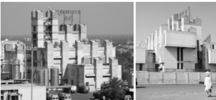
Figure 2. Mehsana Dairy complex with its structural banding and rhythmic ventilation shafts. Photographs by the author.
