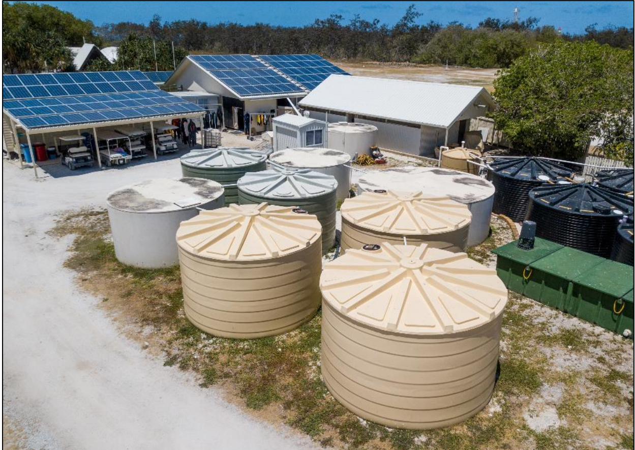
Figure 2. The desalination plant is housed in the shed with the white roof. The freshwater storage tanks in the foreground hold more than twice the eco-resort's daily needs and can supply the eco-resort on cloudy days instead of operating the desalination plant. Note the electric golf buggies used by staff for getting around the island.
