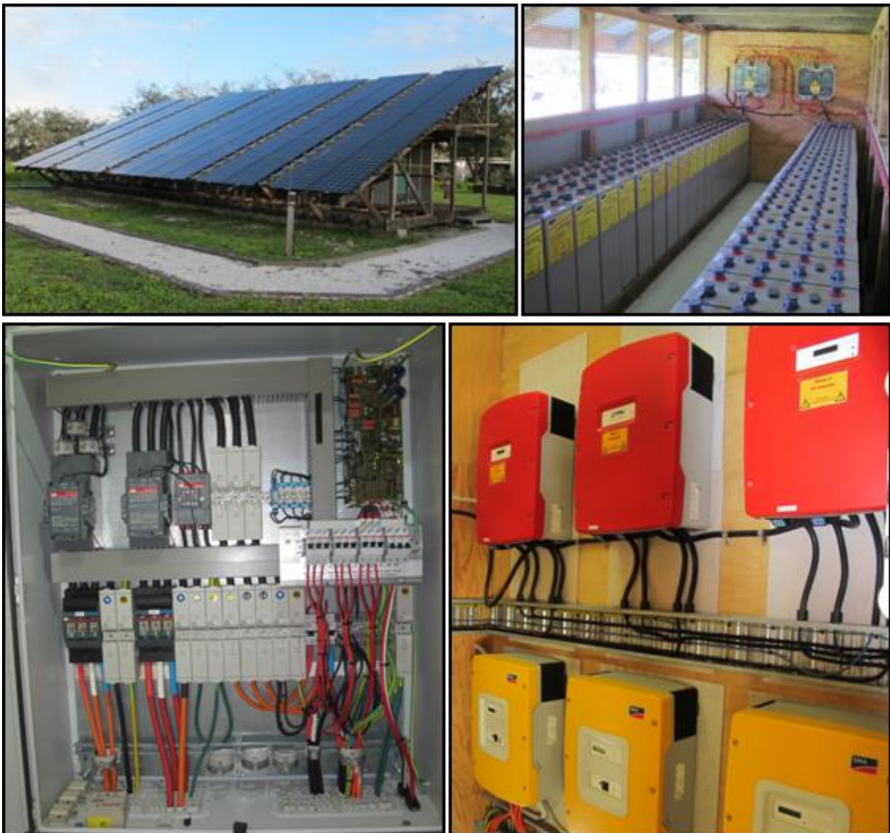
Figure 4. Clockwise from top left. The HSP station soon after it was commissioned in 2008, with the green diesel generator just visible under the solar panels; lead-acid battery banks; the three inverters (red boxes) serving the solar panels, and three inverters (yellow boxes) serving one of the battery banks; and the inside of the multi-cluster control box.
