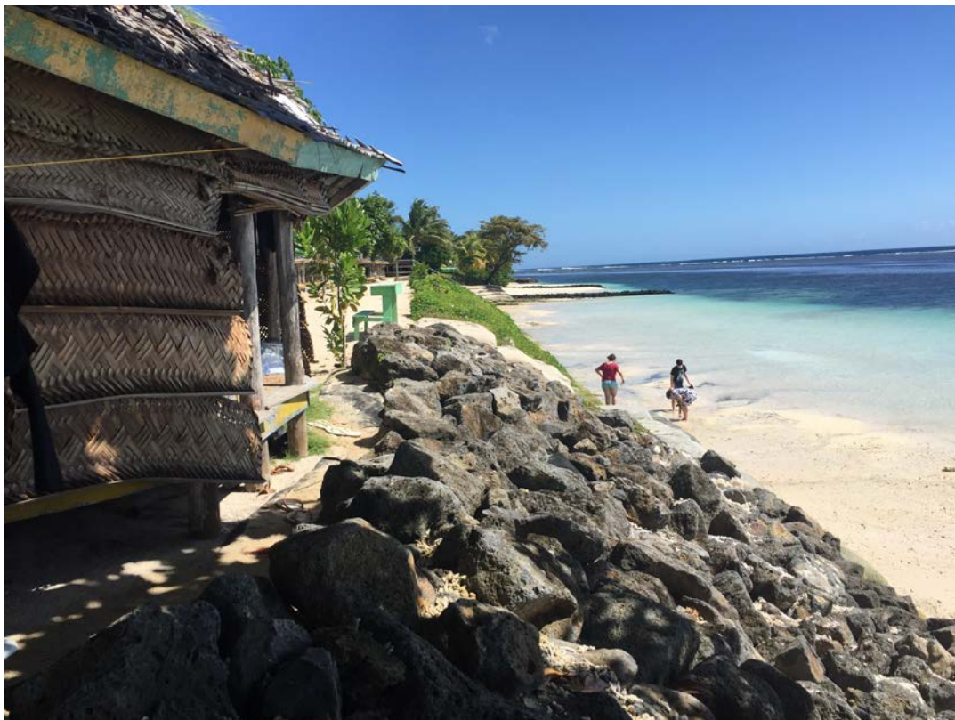
Figure 3. Hard infrastructure (rockwalls) in one of the tourist resorts in Savai'i Island (Samoa) next to sandbags and planted coastal vegetation.
