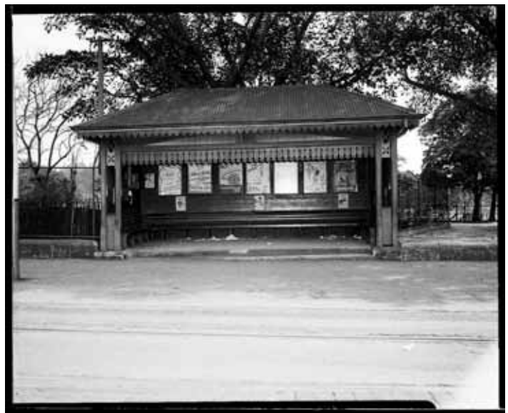
Figure 1. Site of Assault. Tram shelter on City Road. Details unknown.
