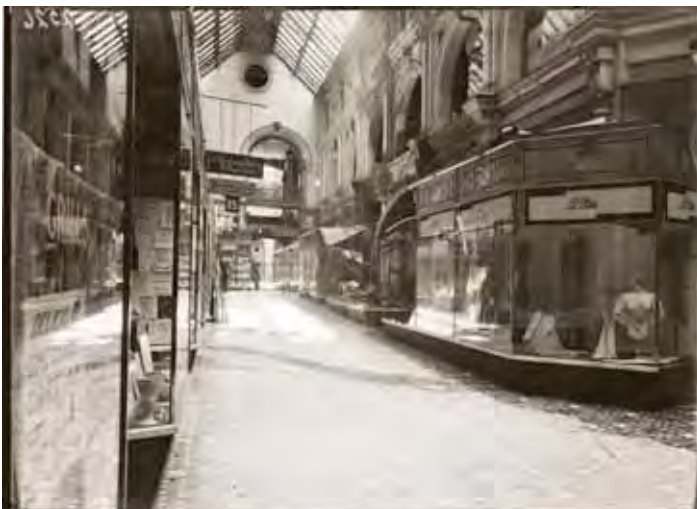
Figure 3. The aftermath of a shopfront fire in the Sydney Arcade around 1937. Details unknown.
