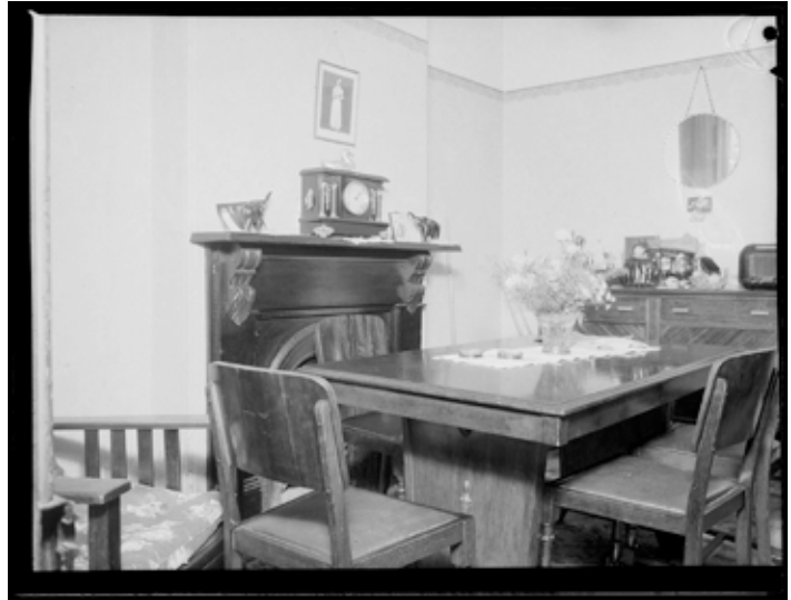
Figure 6. Interior of dining room at a house in Great Buckingham Street.
