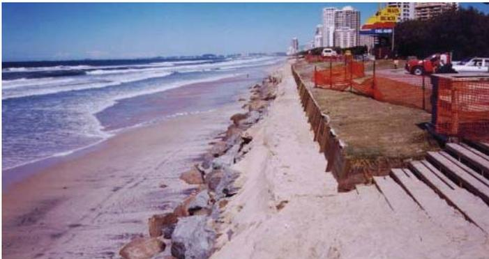
Figure 4. Beach profile at Narrowneck in 1996, before artificial reef construction (Source: GCCC)
