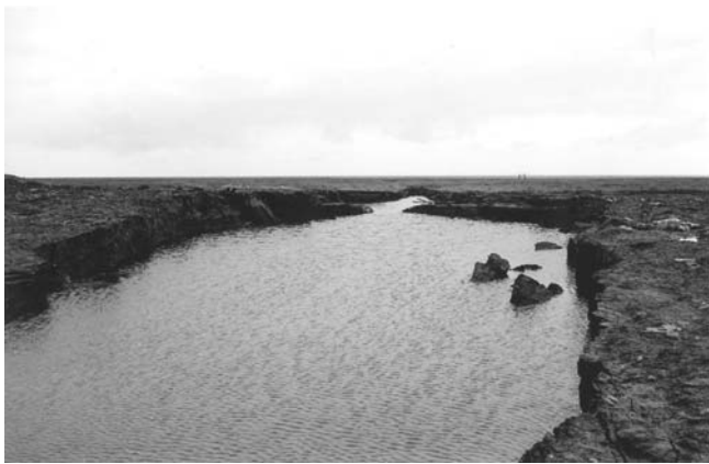
Figure 7. A seaward view of the channel within Breach 1, two months after the initiation of the managed realignment scheme.
