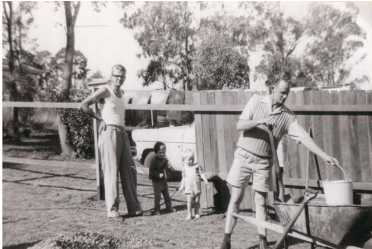
Building fences, Seven Hills 1962 (Karskens family collection)
