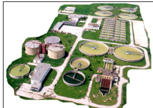
Image: Wastewater treatment plant (GCCM 2006)
