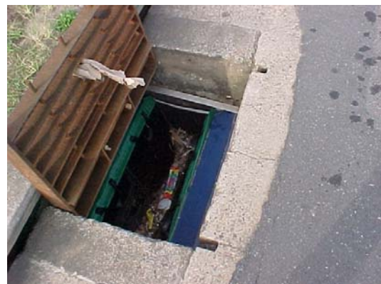
Image: Gully Pit Device – Lawrence Drive
