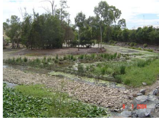
Image: Constructed Wetland – Waterbird Park Sedimentation Lake
