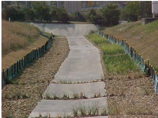
Image: Bio-retention System – Spencer Road
