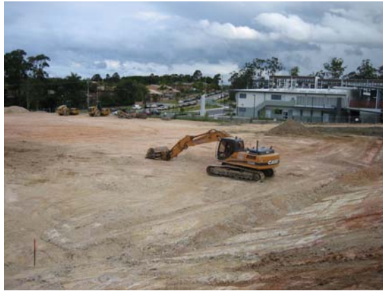
Smart Water Research Facility excavations
