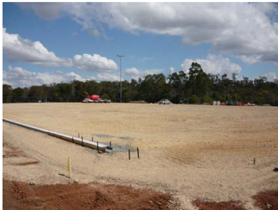
Tennis Centre excavations
