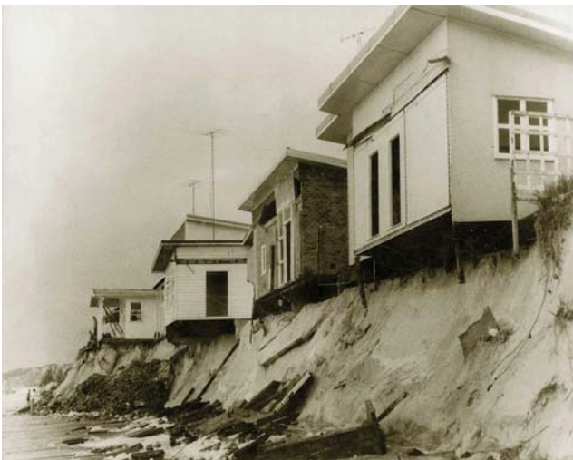
Figure 1 – Structural damage caused by Cyclonic Activity, Mermaid Beach 1967.
