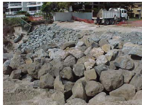
Figure 3, 4 & 5 – Boulder Wall construction at Seashell Avenue Street End, Mermaid Beach
